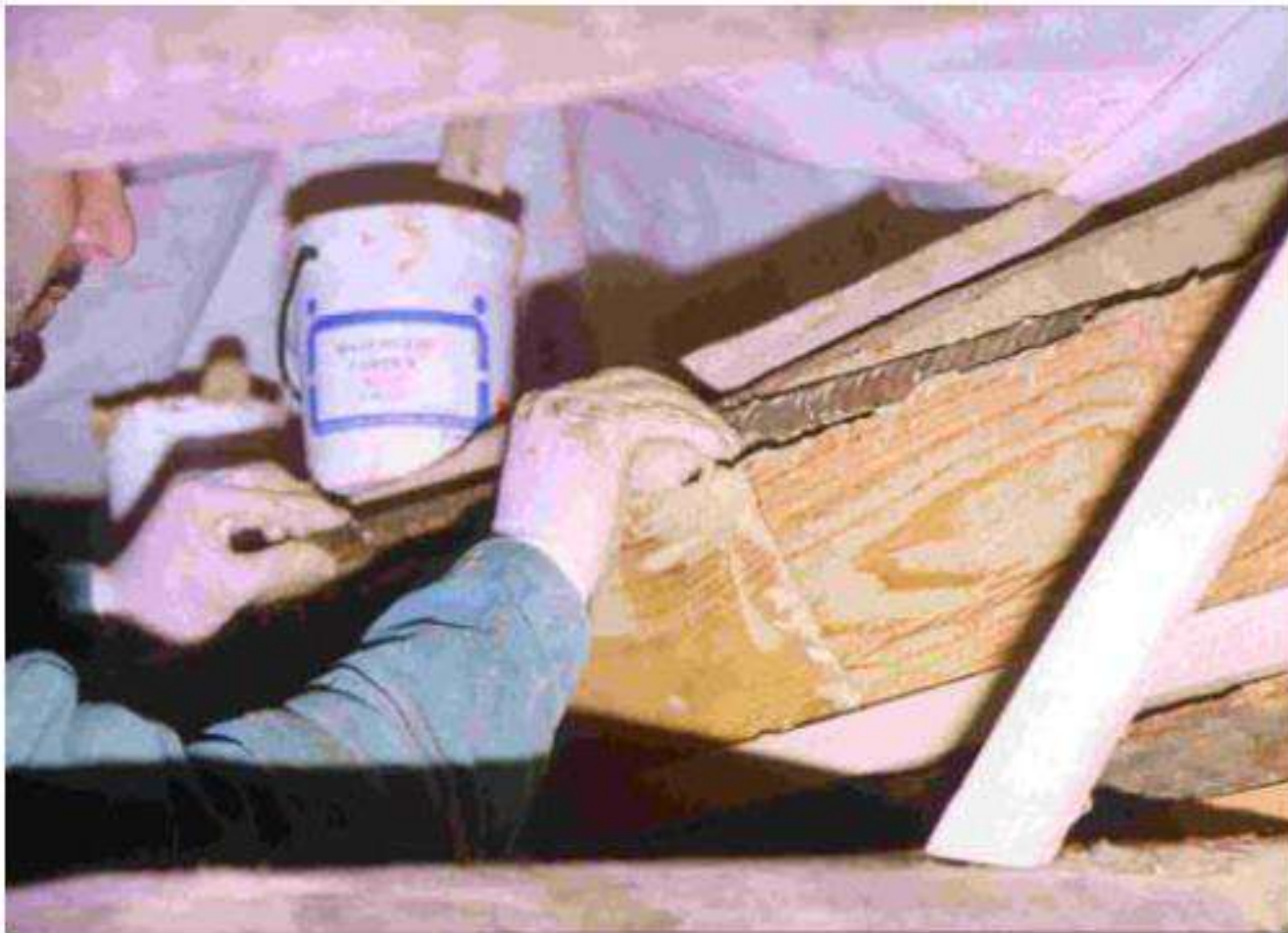
Partially filling of the grooves with adhesive
