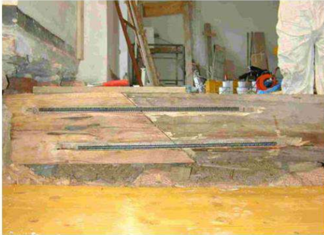
Linking grooves between integration and original timber
