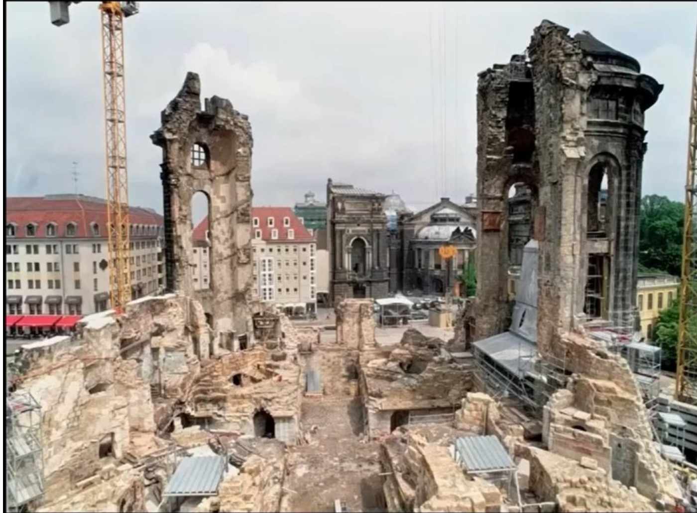
The Church of Our Lady after clearance of site, beginning of reconstruction work
