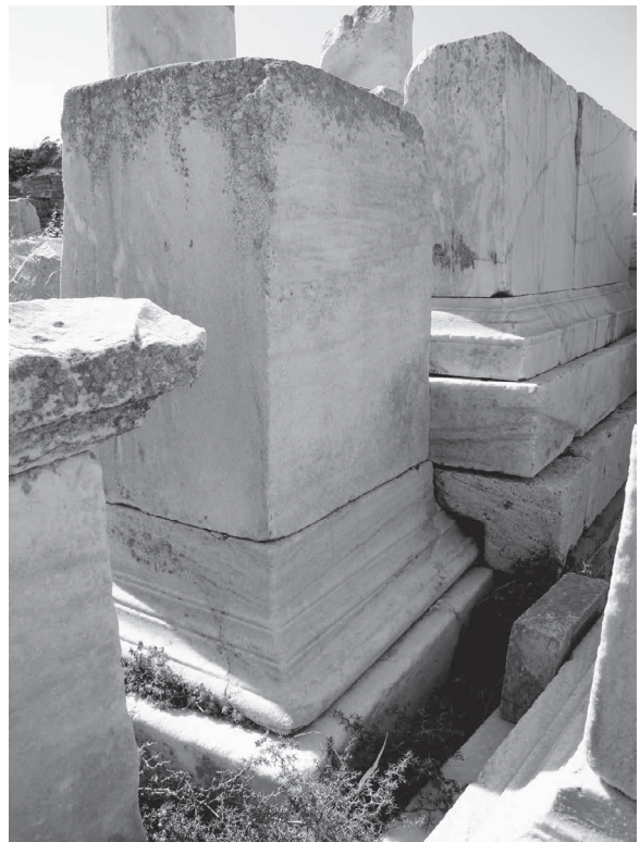
Fig. 18. Detail of the foundation course of the orthostate base for the statues of Krateros and Prince Antiochos Philopator, showing where the orthostate base overlaps the square base for the statue of Zeuxis of Smyrna ( foreground ) (S. Dillon).
