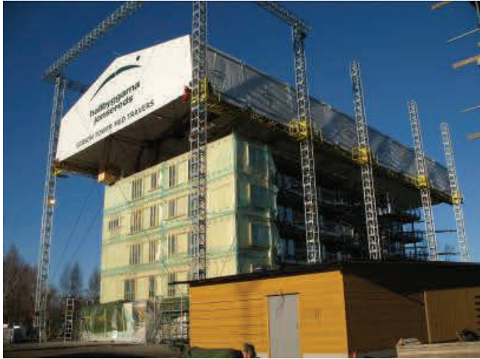
Figure 10 Eight-Story Building Under Construction Protected by a Tent
