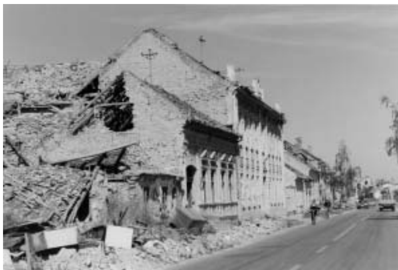
War-damaged homes, Vukovar, Croatia, September 1992
