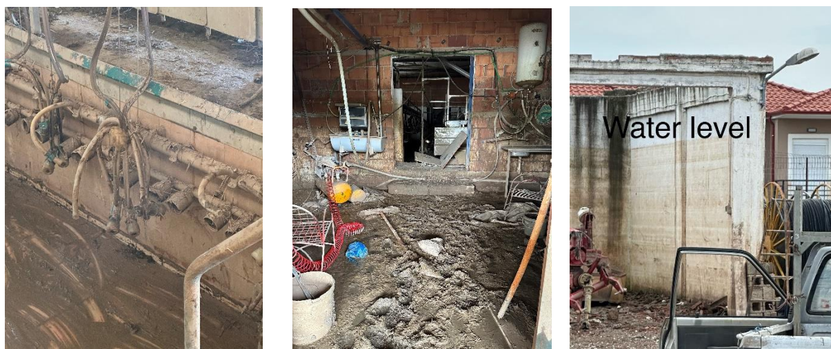
Figure 13: Total loss of milking machinery
