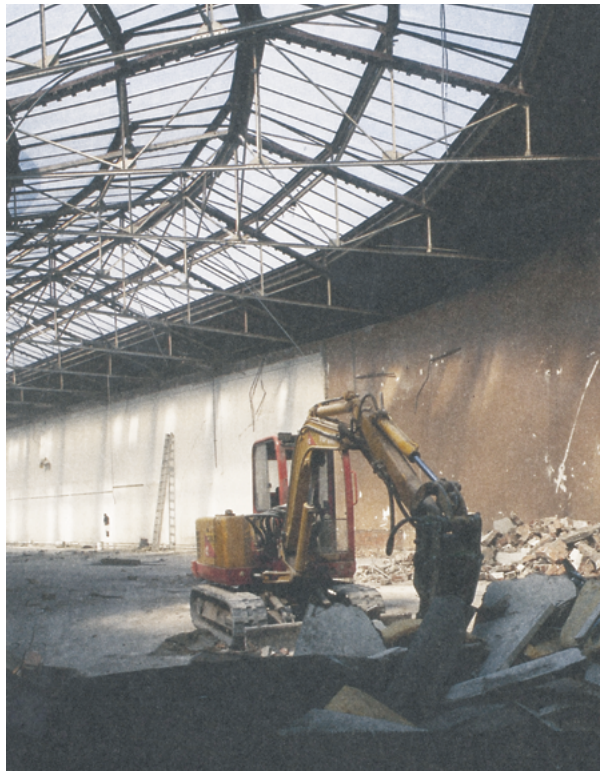
Sculpture hall, construction works, 1996.
