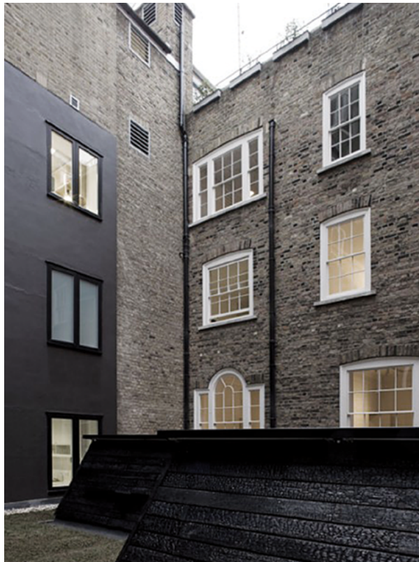
Raven Row, the skylights clad in charred wood in the courtyard visible from the gallery.
