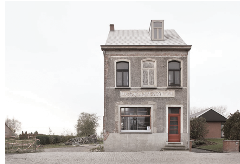
The street façade viewing the Koppenberg.
