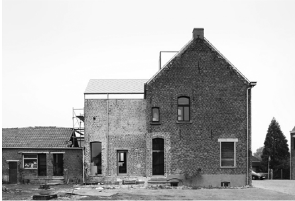
The Rot-Ellen-Berg under (re)construction, 2009.
