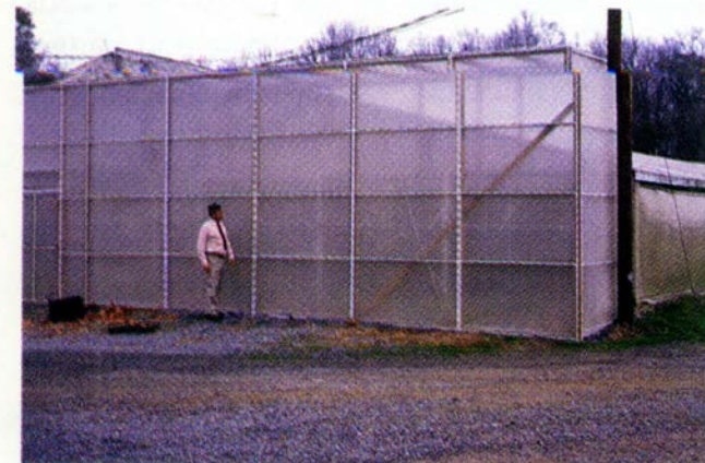
Fig. 10. Thrips exclusion screening. Porchlike addition at end of greenhouse provides increased surface area, which is necessary to compensate for reduced air flow.
