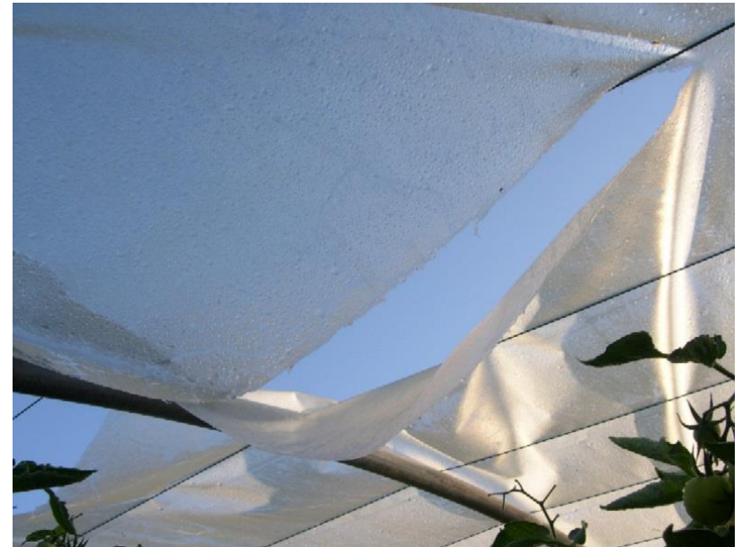
Typical ageing coming from film contact with the frame (wires)
