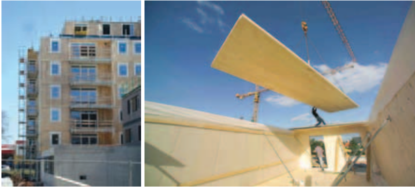
Figures 2.3 Prefabricated Engineered Timber Buildings Store Carbon
