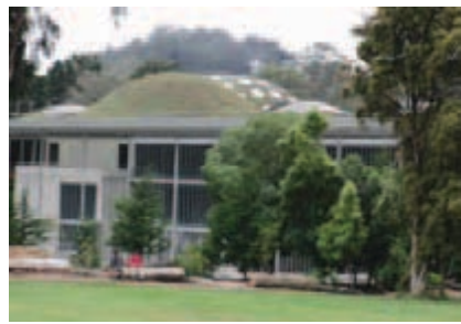
Grass Roofing: Science Museum, San Francisco
