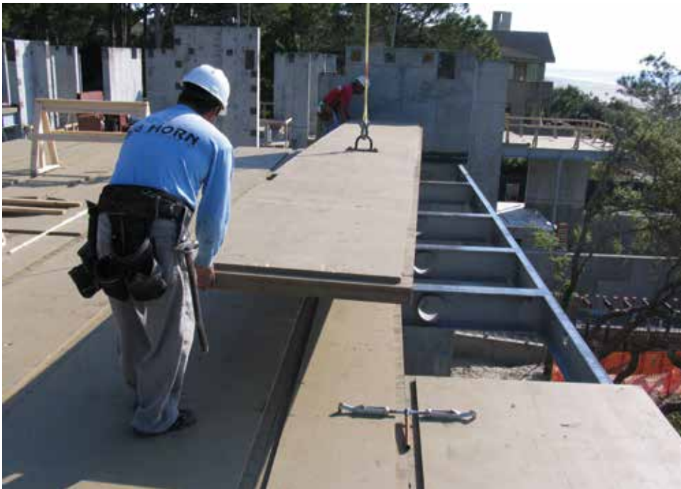
Figure 7 Lifting and handling of CLT elements in an hybrid structure, in the United States (courtesy of Binderholz)
