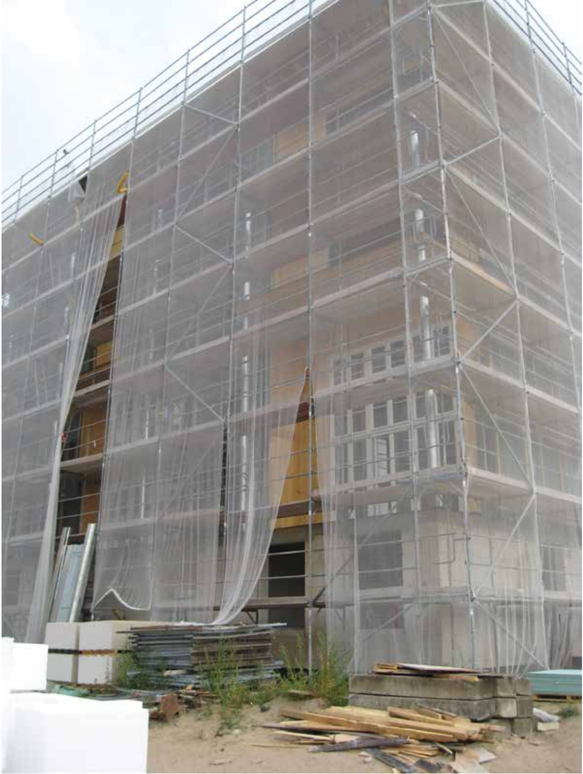
Figure 59 Use of a water-proof tarpaulin outside scaffoldings – Germany
