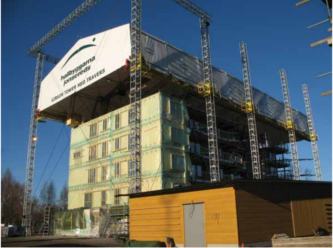
Figure 60 Use of an adjustable tent – Sweden
