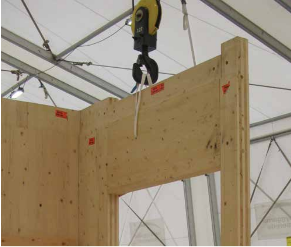
Figure 21 Lifting sling without support (with hole)
