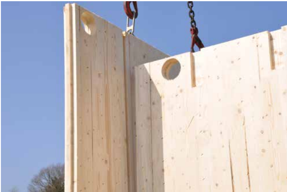
Figure 25 Screwed anchor
