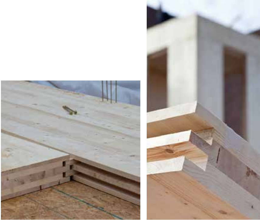
Figure 7 Double internal splines (Courtesy of Kevin Meechan and U.S. WoodWorks)
