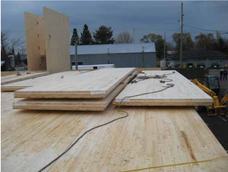
Figure 57 CLT slabs temporarily stored on a floor
