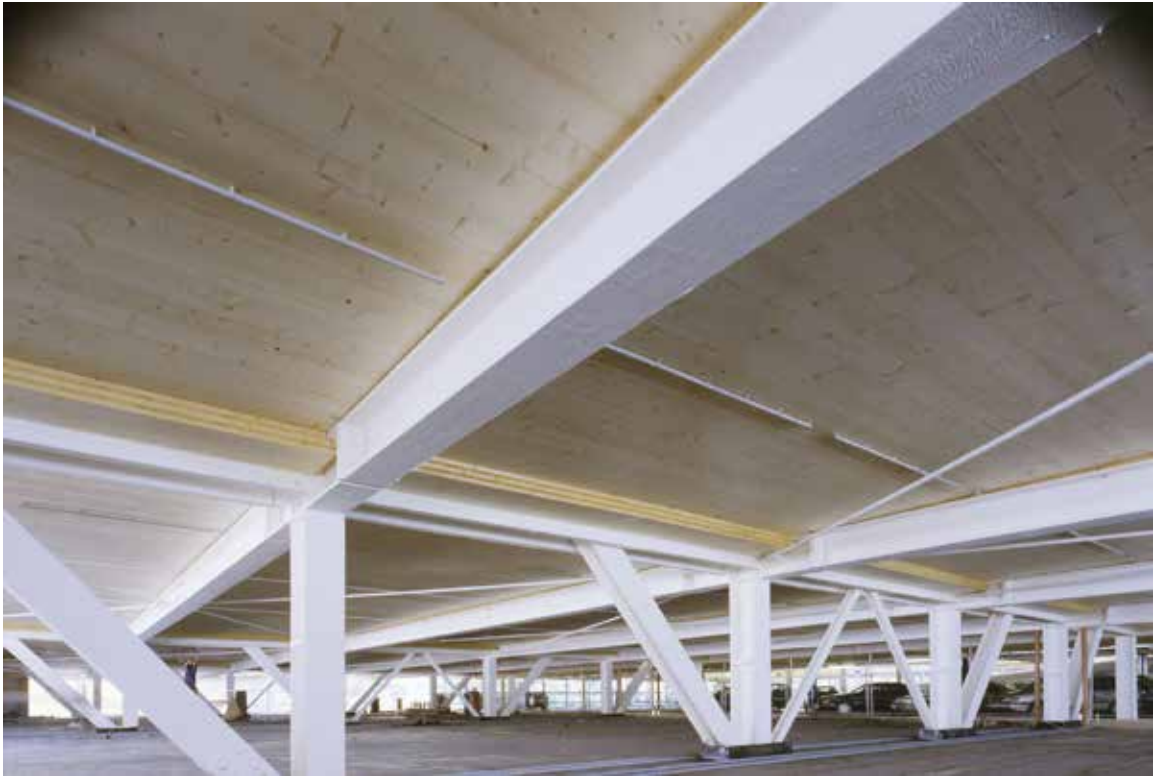
Figure 30 Parking garage in Innsbruck, Austria (courtesy of KLH)
