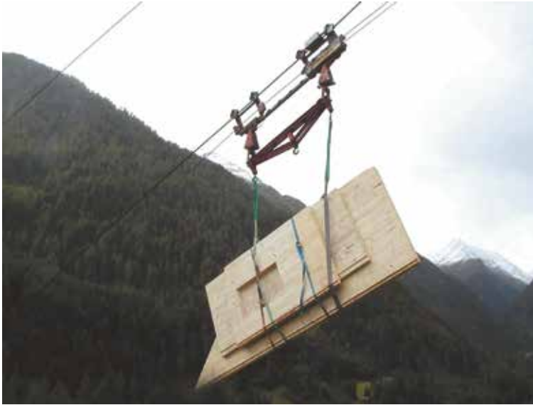
Figure 12 Lifting and handling of CLT elements by cableway (courtesy of KLH)
