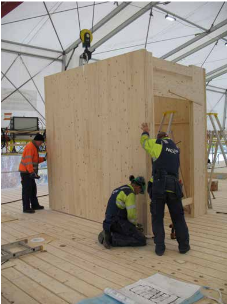
Figure 22 Multi-family building in Växjö, Sweden
