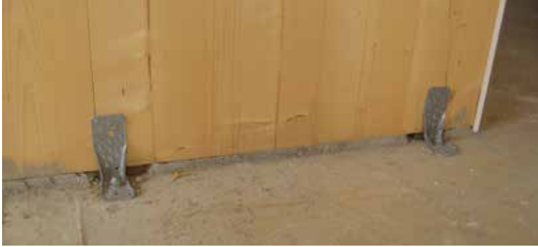
Figure 32 Metal brackets installed on site
