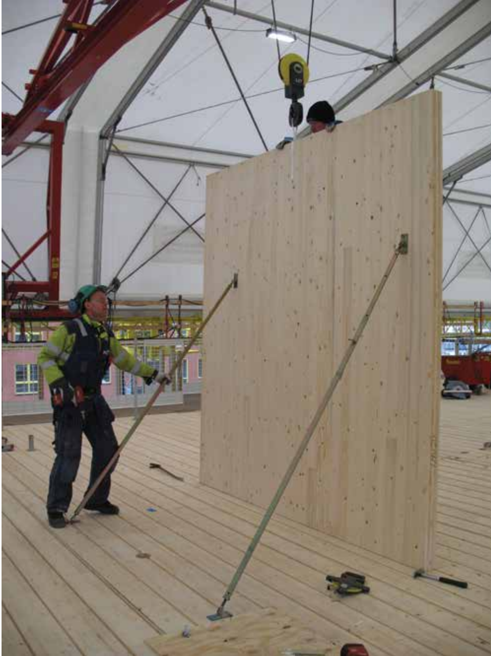
Figure 44 Adjustable shoring for walls
