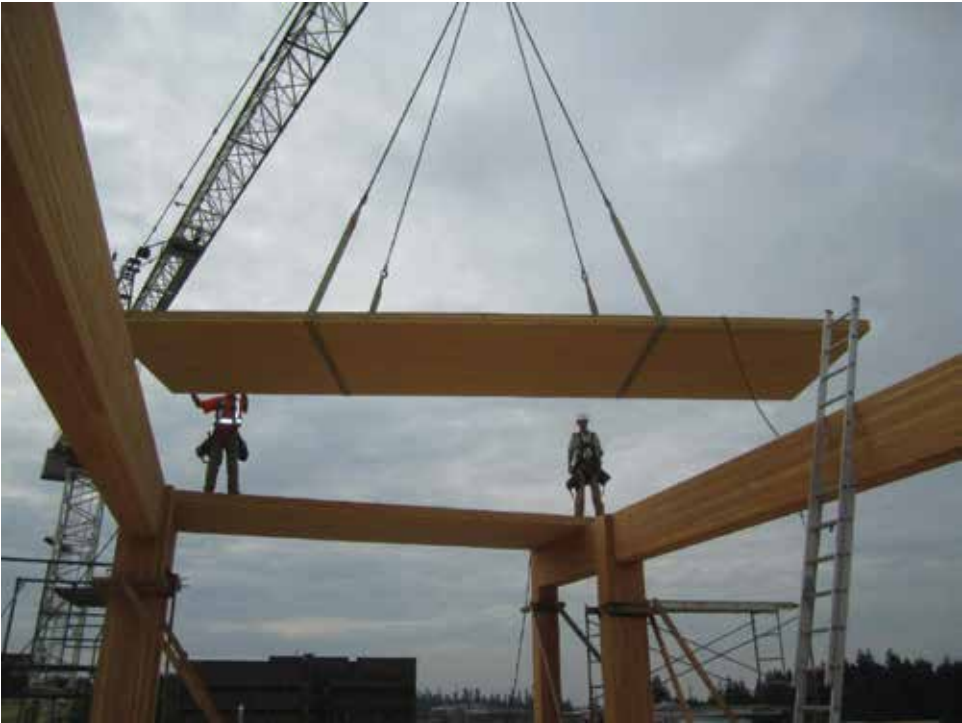
Figure 22 Lifting sling without support (without hole)
