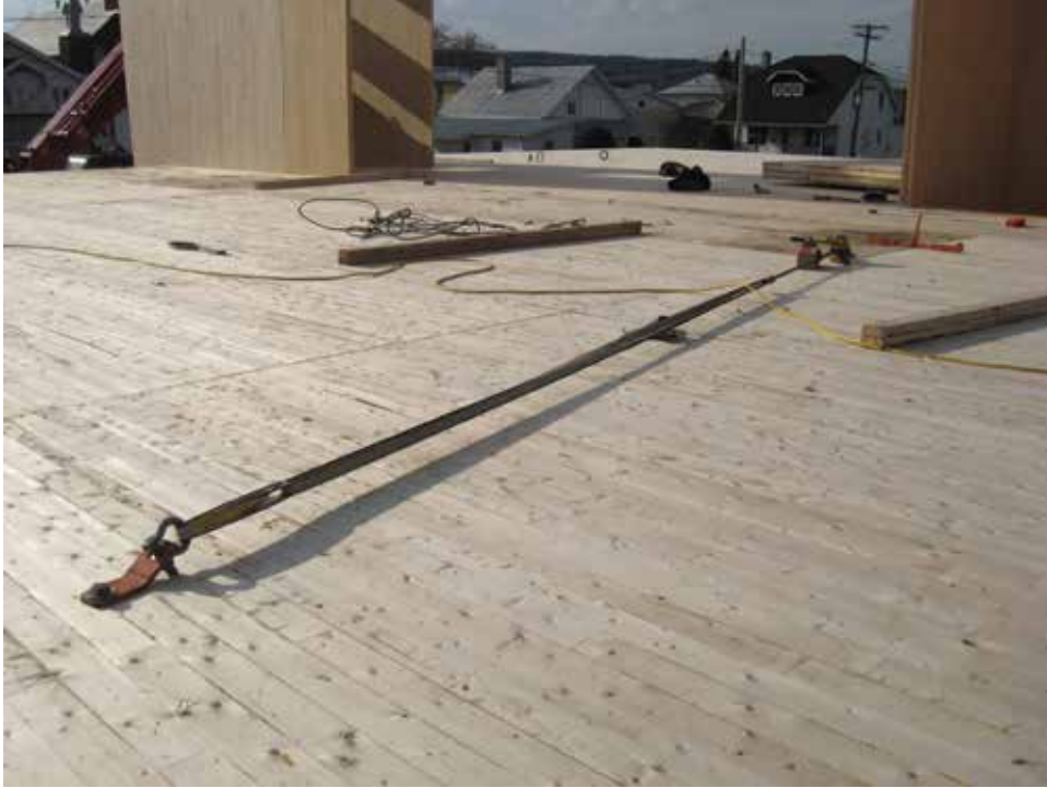
Figure 47 Manual winch used with soft slings
