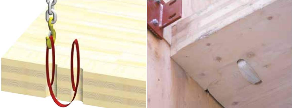
Figure 23 Lifting sling without support (with holes)
