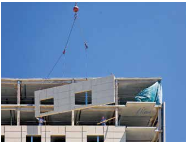
Figure 1 Lifting and handling of precast concrete elements
