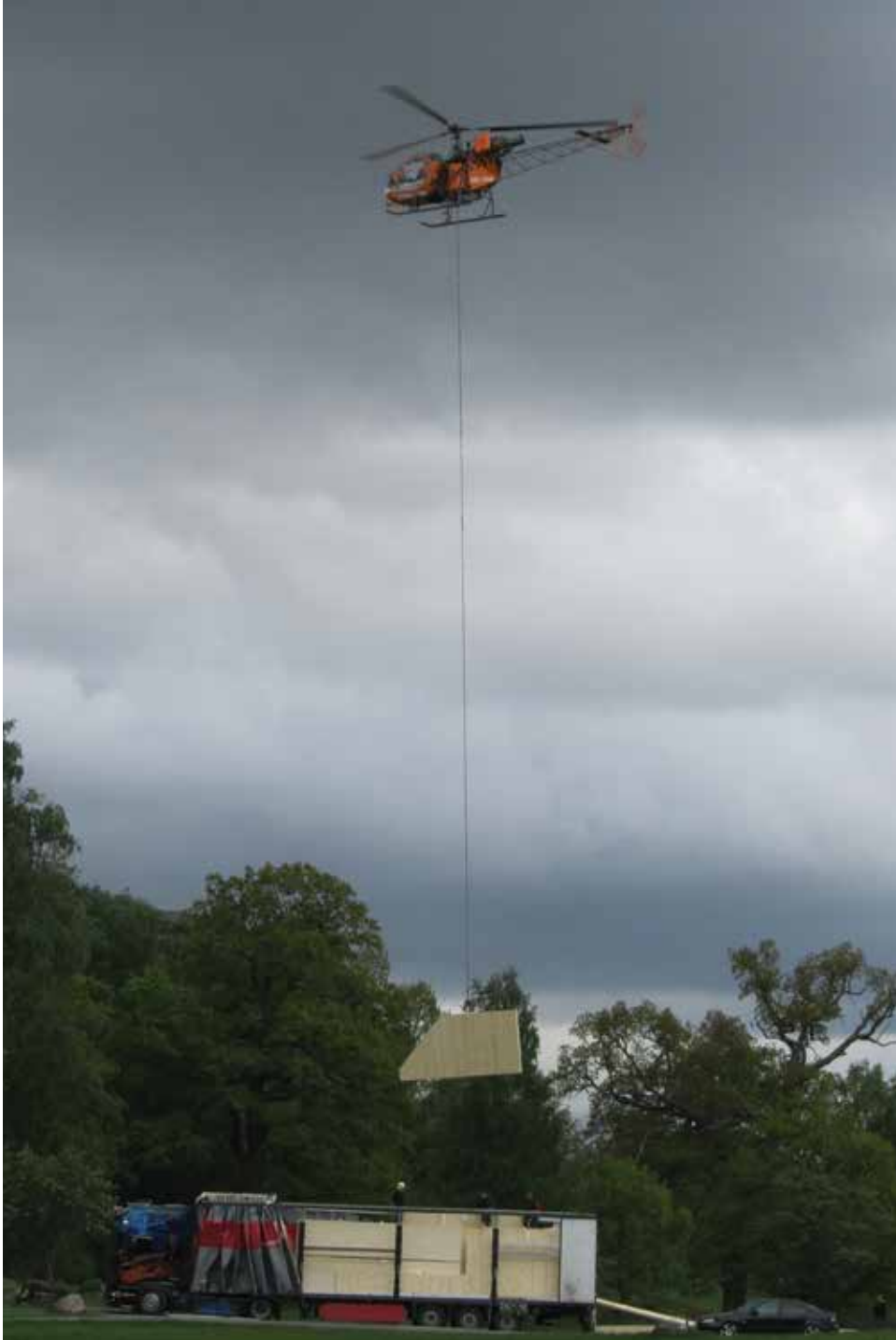
Figure 3 Lifting and handling of CLT elements by helicopter (courtesy of KLH)
