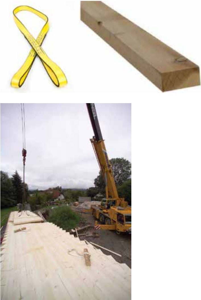
Figure 20 Single lifting sling used with support
