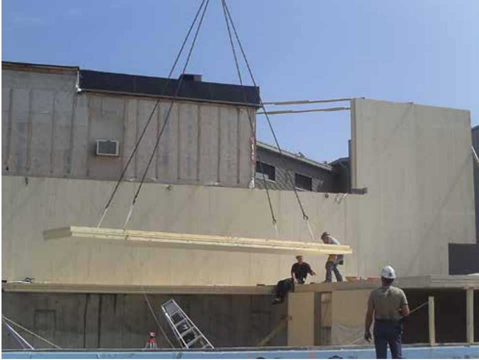
Figure 6 Lifting and handling of CLT elements, in Canada (courtesy of KLH ELEMENT, photo: © Marc Cramer)
