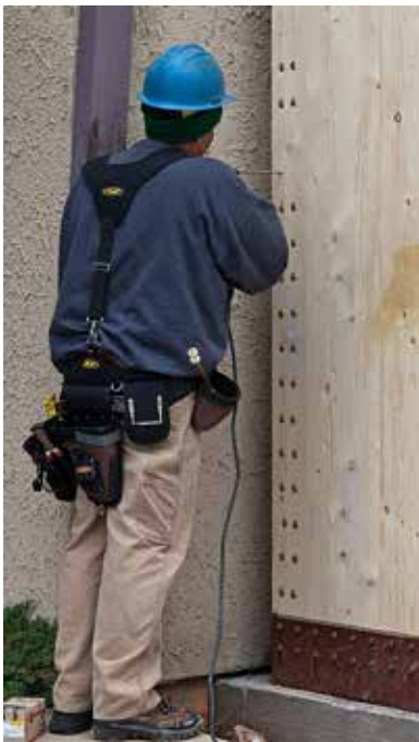
Figure 13 Installation of self-tapping screws from the exterior (courtesy of U.S. WoodWorks)
