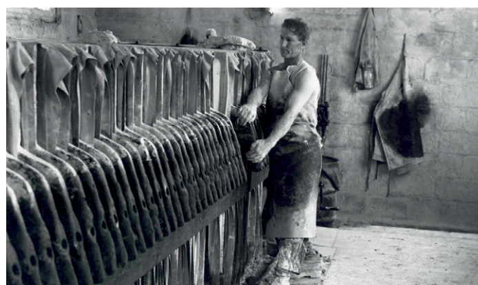
Figure 2: Filter press in operation from around 1900. (Wheal Martyn Museum, St Austell, UK)
