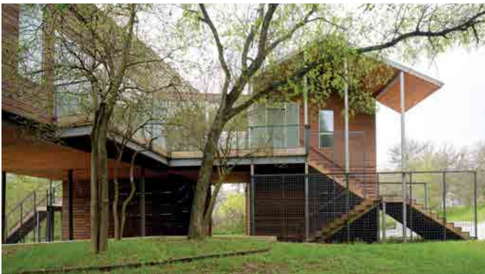
Guadalupe River House - Side view - Storage rooms are situated on the ground floor, less vulnerable in case of flood.
