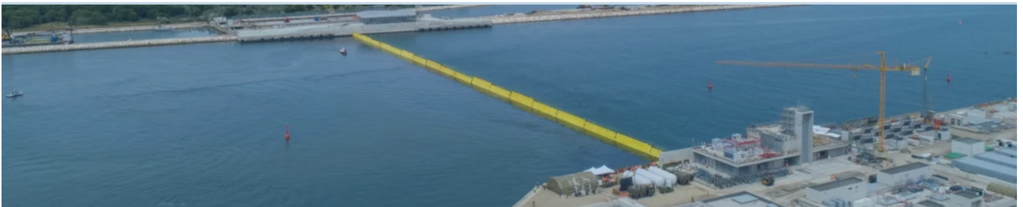
the engineering solution to combat "acqua alta"
