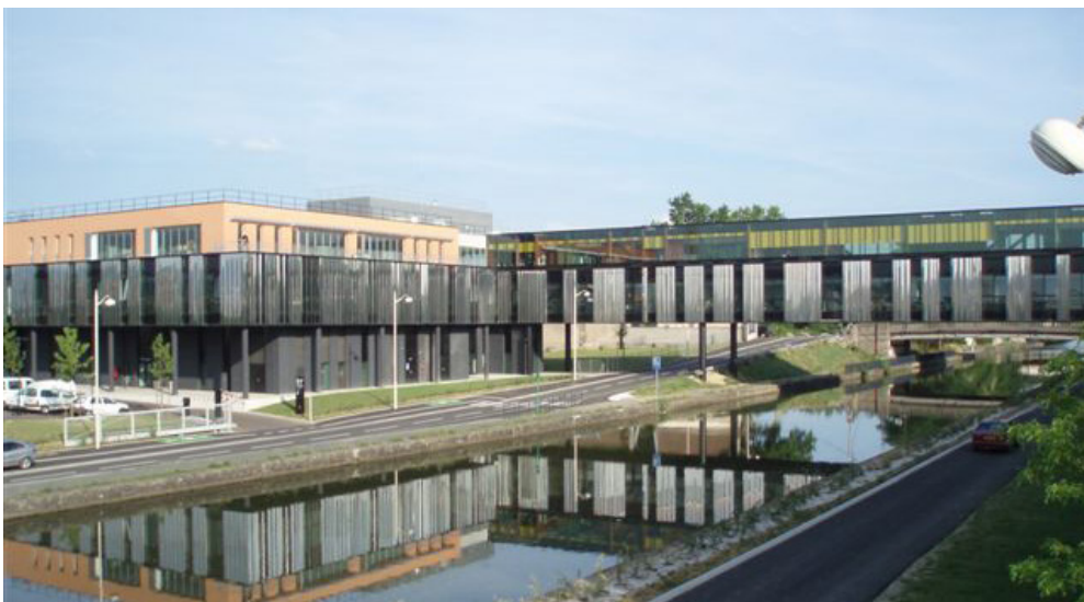
IRR Nancy - bridge view - A bridge cross the canal 8m above it. This enable people to access the building from both sides of the canal.
