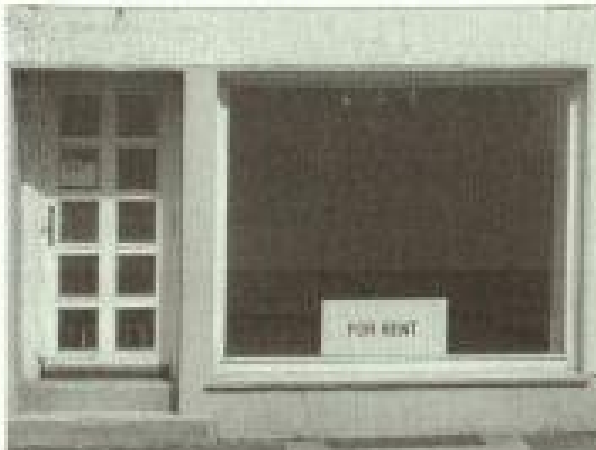
Fig. 34: Vacancy may indicate that a structure is not fit for purpose.
