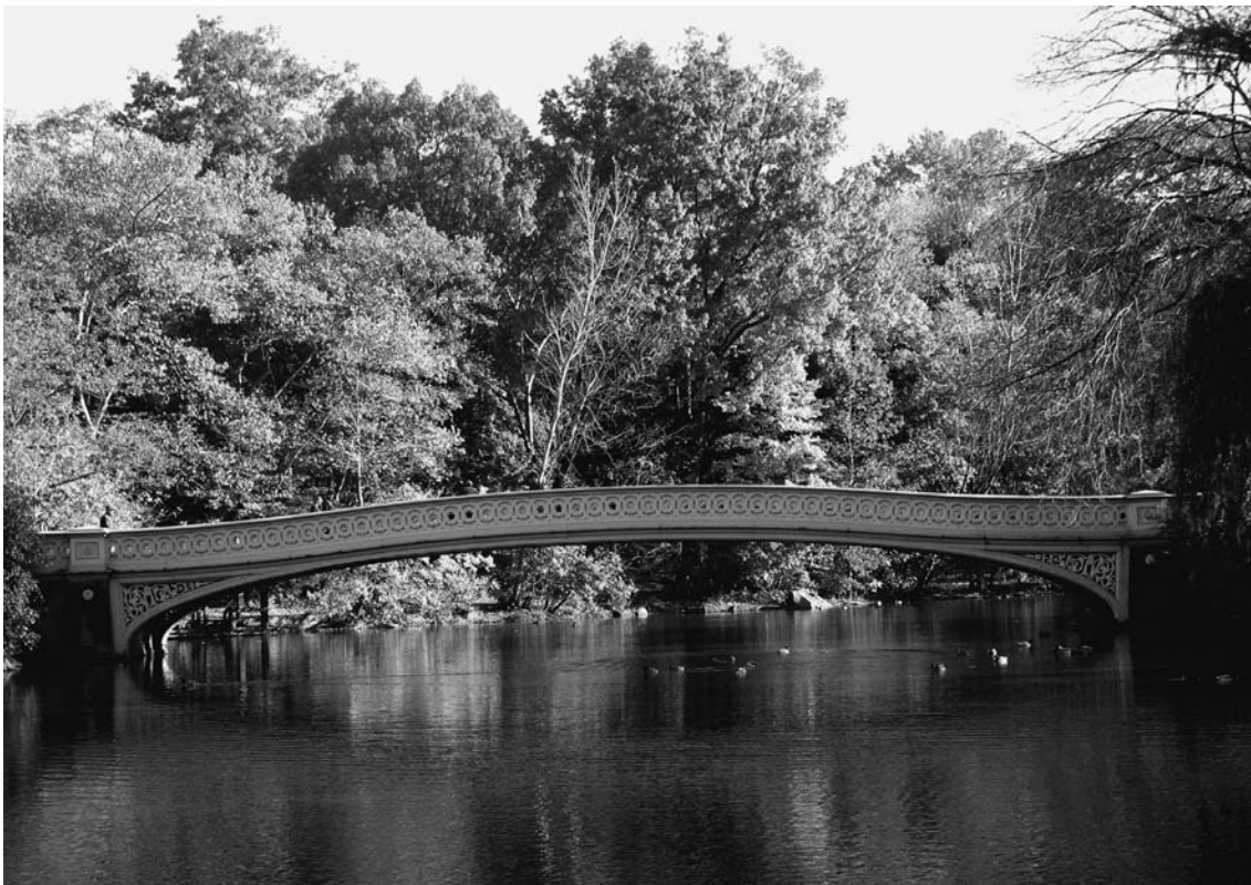
8.2 Bridge on lake, Central Park
